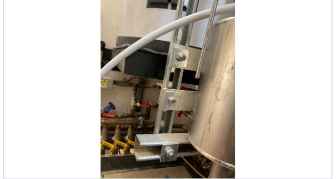
SITE PHOTOGRAPH GP08
