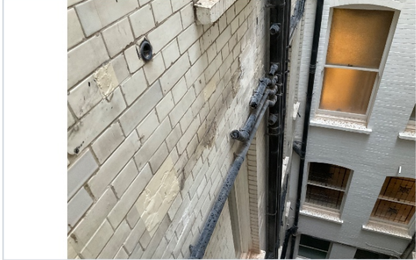
SITE PHOTOGRAPH GP02
